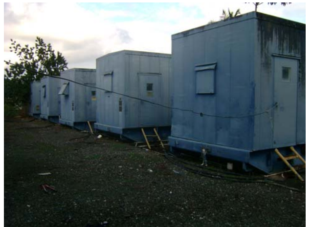
12 Cylinder self contained units, including 480VAC Motor control center, 4160VAC Switchgear, Battery charger, diesel air compressor, engine control and protection panel
