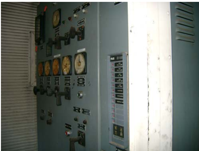
12 Cylinder self contained units, including 480VAC Motor control center, 4160VAC Switchgear, Battery charger, diesel air compressor, engine control and protection panel
